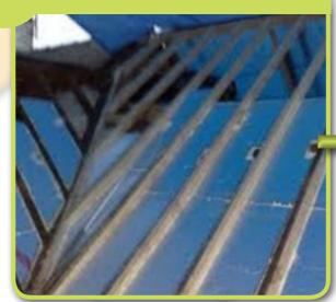
**Step 6** New felt is fitted to the roof
